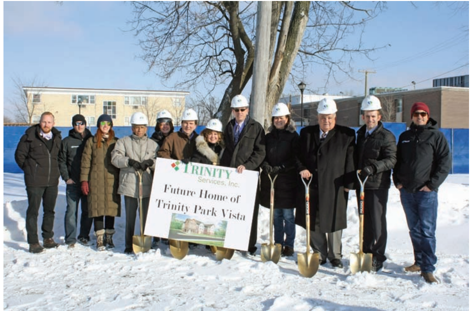
Representatives from Trinity Services, Inc.; the City of Northlake; Worn Jerabek Wiltse Architects, P.C.; Brush Hill Development; the Illinois Housing Development Authority; and Synergy Construction Group celebrate the groundbreaking of Trinity Park Vista Jan. 16 in Northlake.
